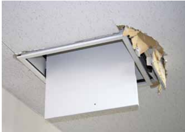
A smoke vent, which should open only in case of fire, was malfunctioning due to the quake.
