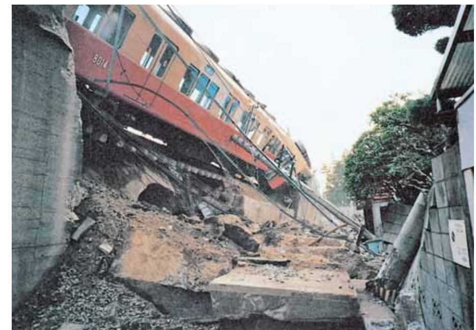
Railways (Japan Railways, Hankyu, Hanshin, and Sanyo) had tremendous damage, including the collapse of stations and train derailments. Moreover, due to the collapse of the underground Daikai Station on the Kobe Rapid Transit-Railway line, a national expressway above the station caved in. Although alternative transportation was provided immediately after the quake in collaboration with the railway companies by using buses, there were large-scale traffic jams in many parts of the city.
