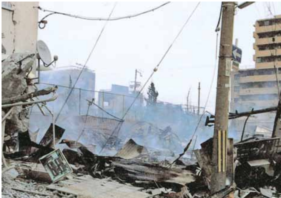
Nagata Ward area had a huge fire, creating a tragic situation similar to war damage. It is said that the huge fire was caused by electrical leakage when electricity was temporarily restored after the power shortage. Sufficient fire extinguishing activities could not be conducted due to the water outage.
