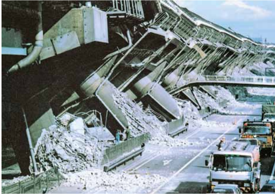
The Hanshin Expressway was closed, because of the 640 meter-long collapse around Fukae-honmachi in Higashinada Ward area, Kobe City which is on the No.3 major Kobe highway. Five bridges collapsed and this caused tremendous traffic jams on neighboring expressways.
