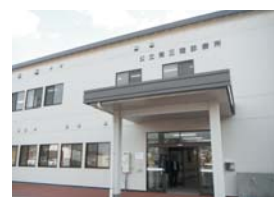
Temporary hospital for secondary medical care (Minamisanriku, Miyagi Prefecture)
